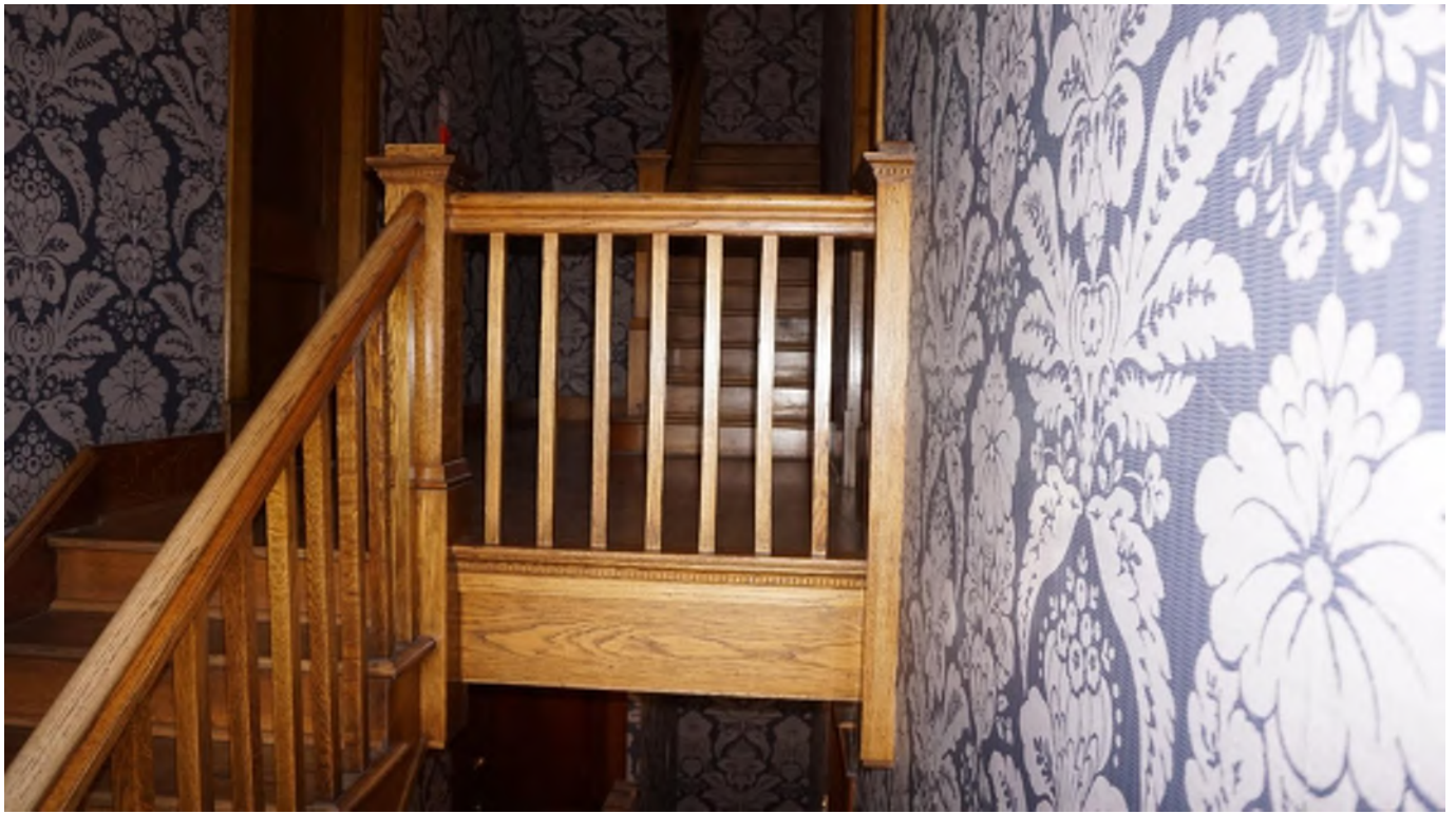
Figure 61 - Wallpaper in Building 904.
