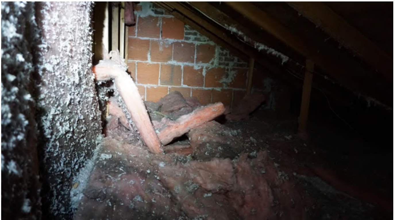
Figure 5 - Example of uninsulated knee-wall sections.
