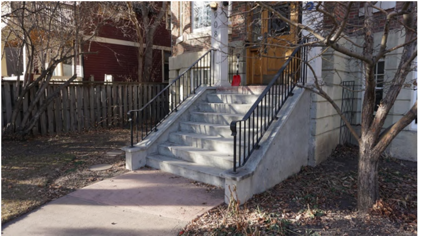
Figure 62 - Concrete sidewalk, steps, and landing
