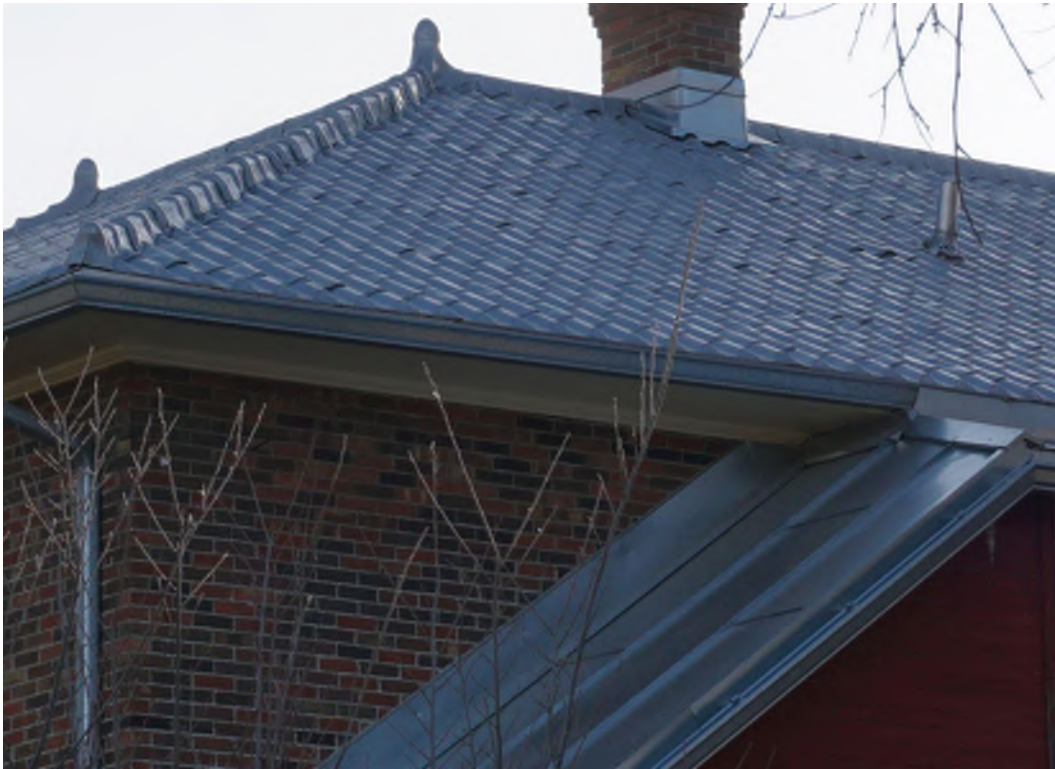
Figure 21 - View of Spanish Tile metal roof shingles.
