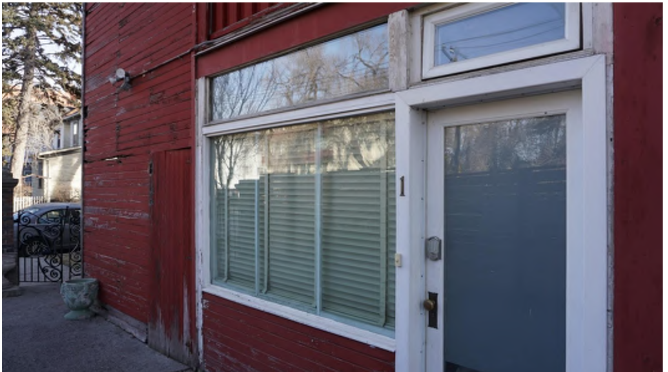
Figure 23 - Exterior security lighting and doorbell.
