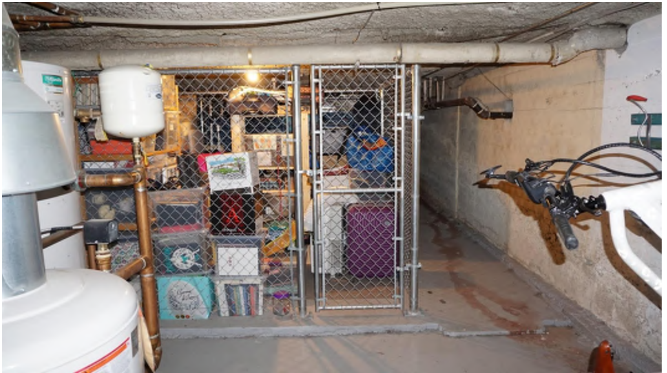
Figure 56 - Chain link storage lockers.
