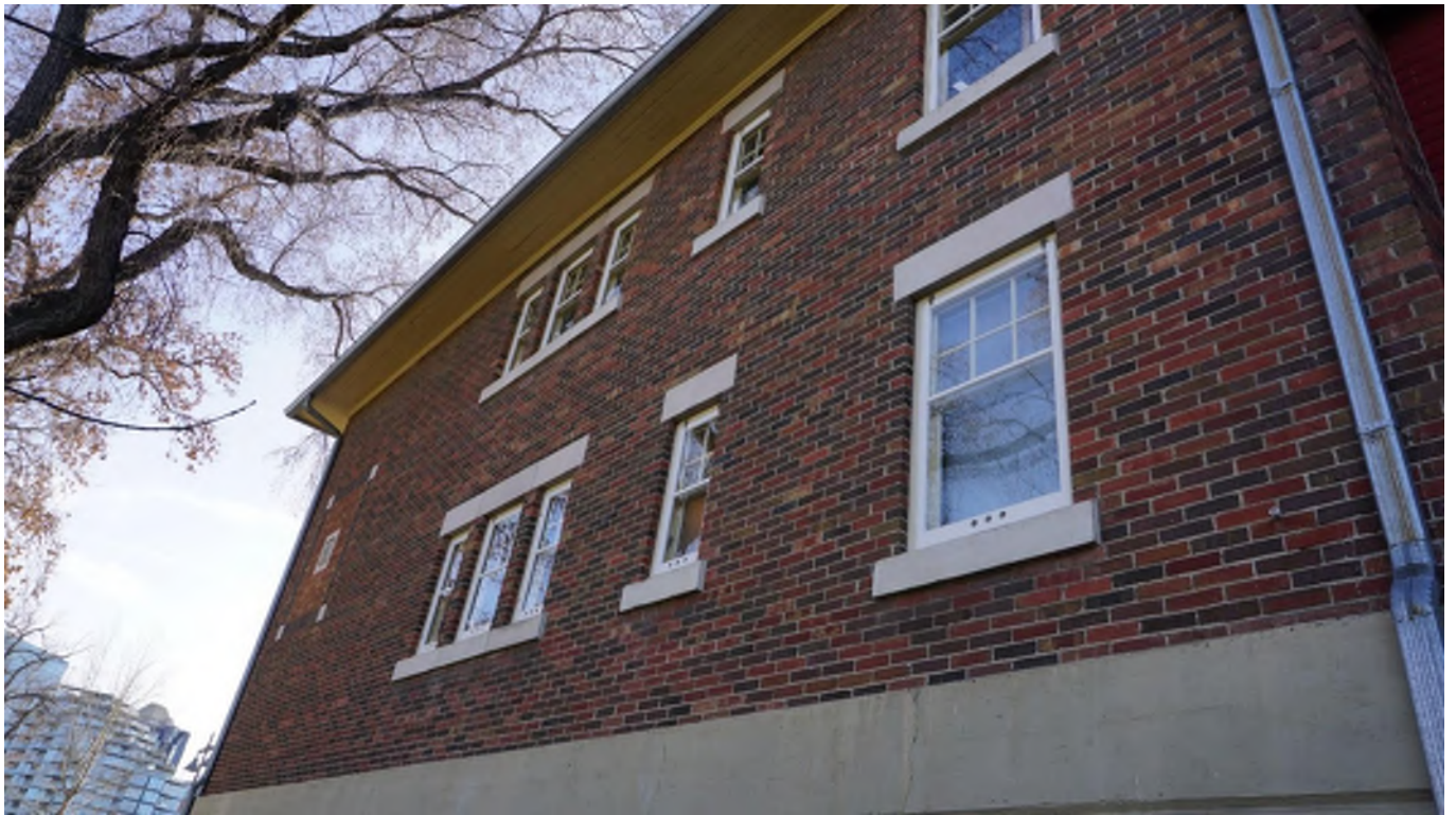
Figure 6 - Example of the general character of the brick facade.
