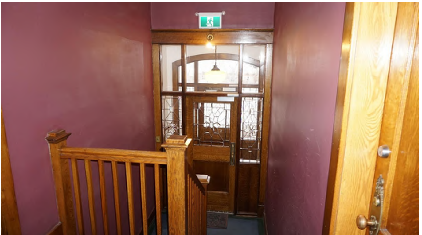
Figure 9 - View of the interior side of the entry door system.
