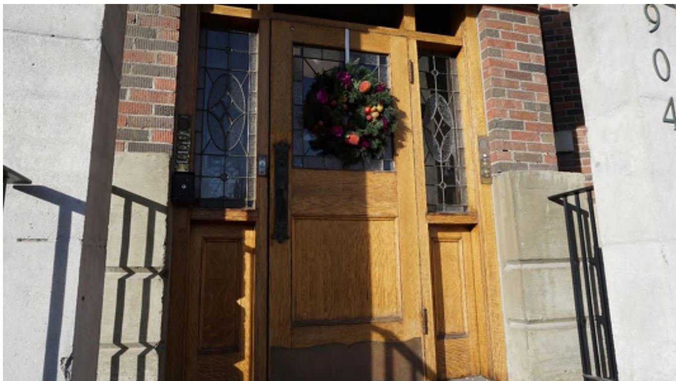
Figure 10 - Exterior view of the original hardwood doors with original hardware.
