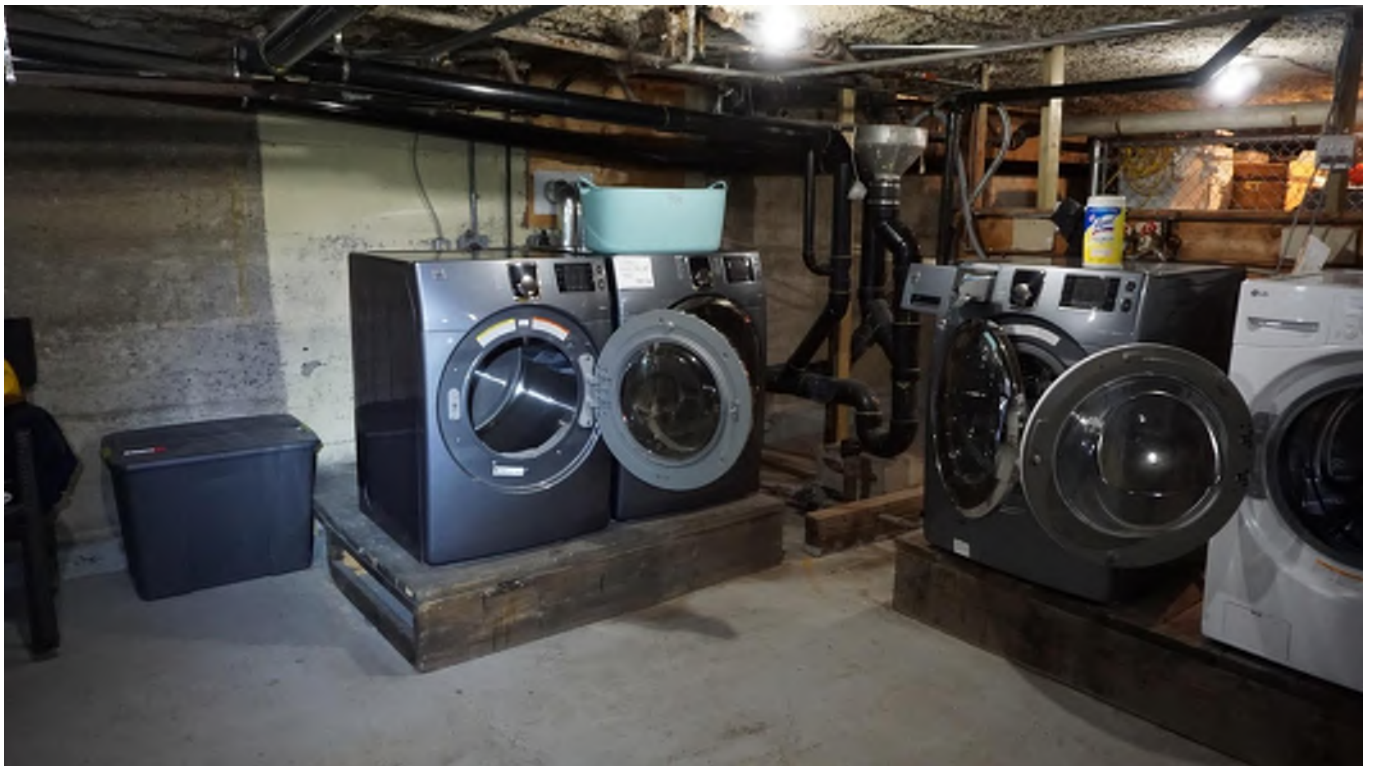
Figure 38 - Various drain lines.
