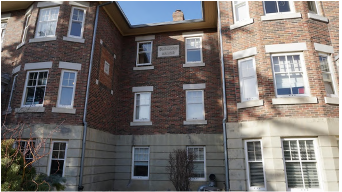
Figure 16 - Typical main building windows.
