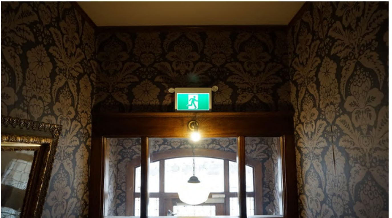
Figure 26 - Pendant and wall mounted fixtures at the front entrance.
