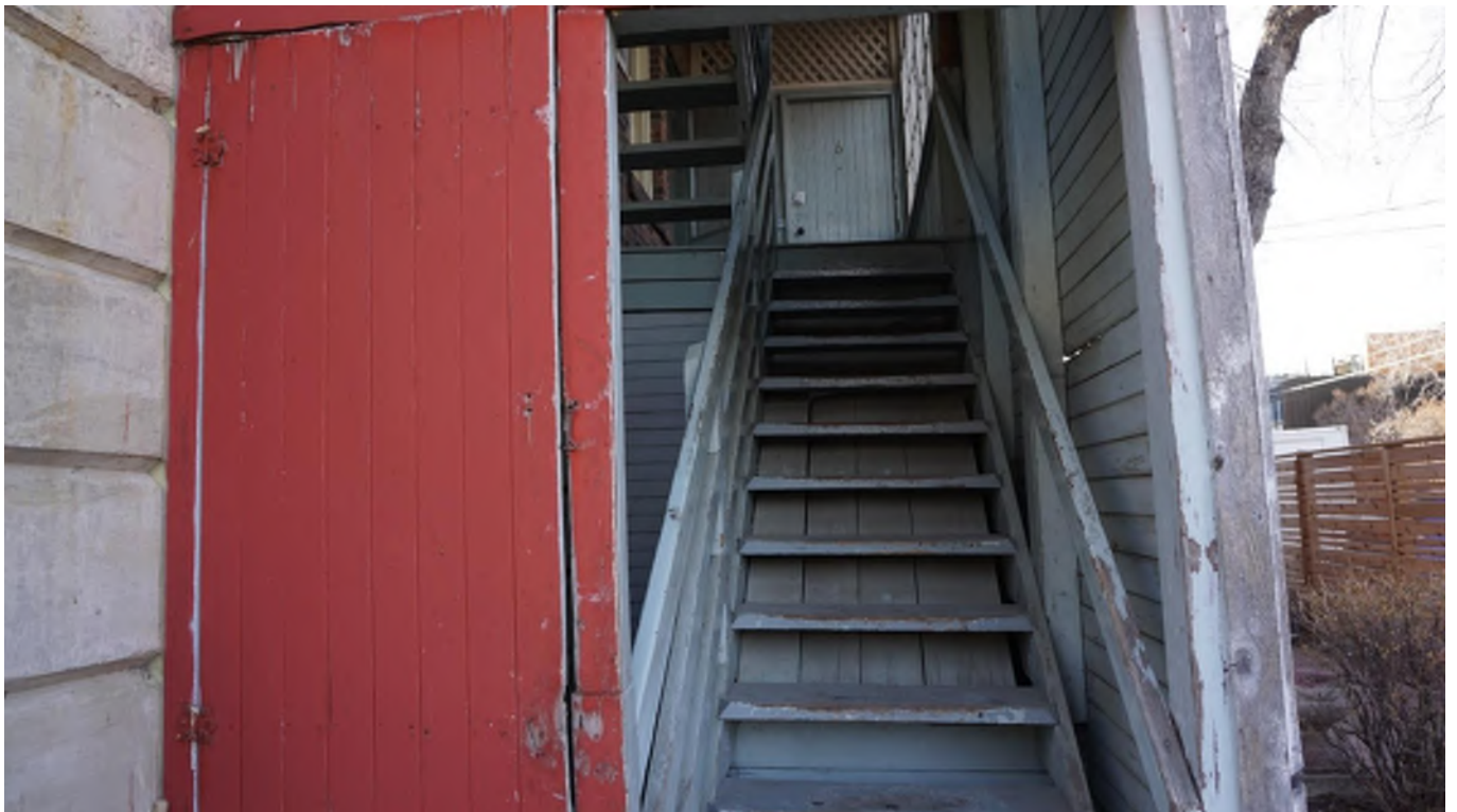
Figure 14 - Example of veranda partition door and safety door for external basement stairwell.
