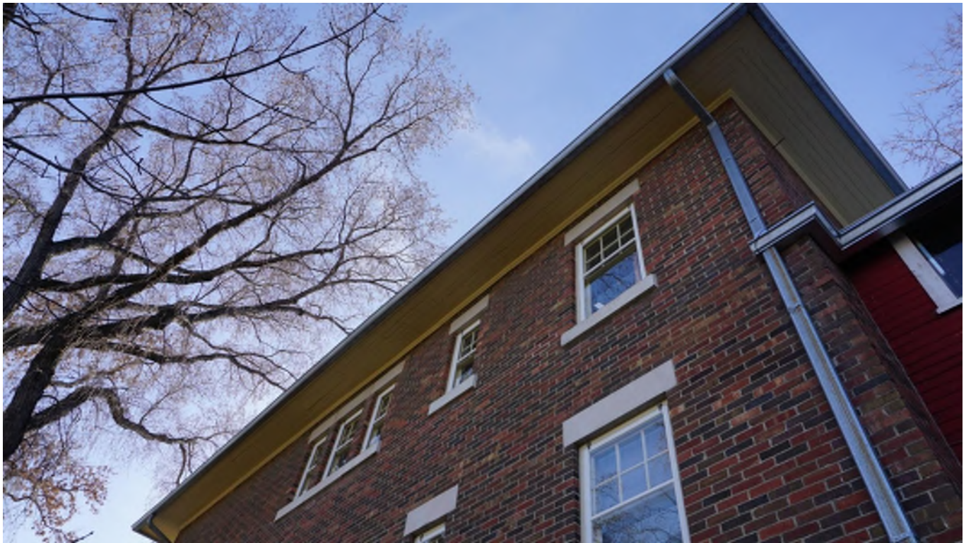
Figure 20 - View of galvanized gutters and downspouts.
