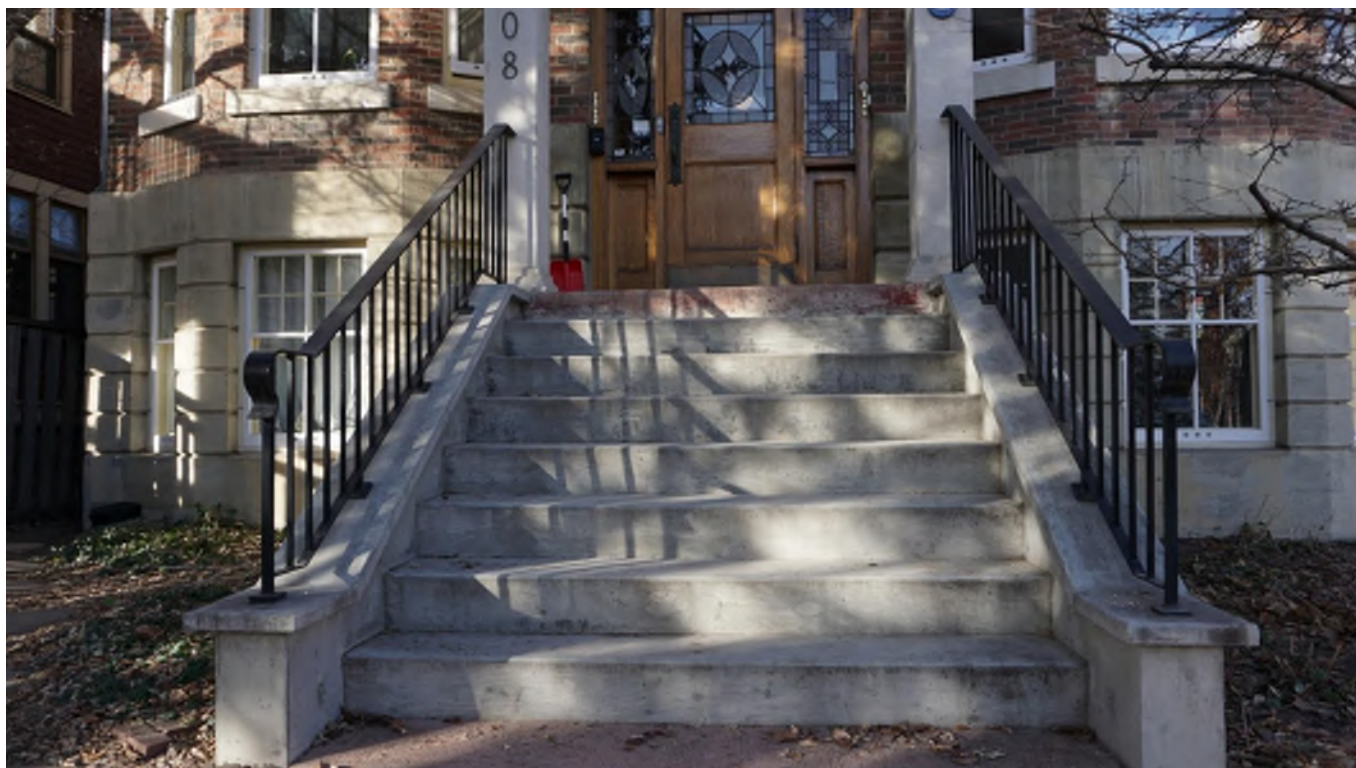
Figure 75 - Wrought iron hand and guard rails.
