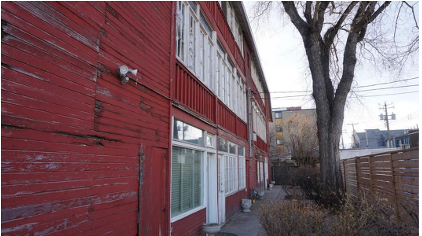
Figure 17 - Example of rear exterior windows on the veranda.
