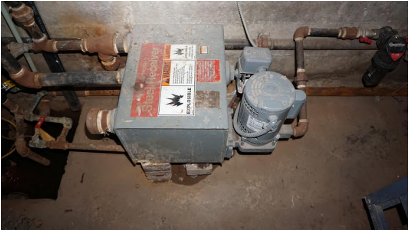
Figure 35 - Condensate system.
