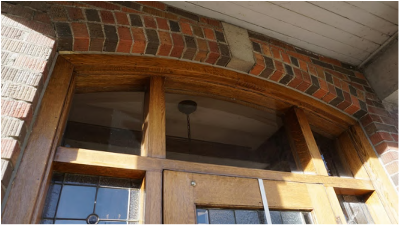
Figure 15 - Example of sealants around the front entrance.
