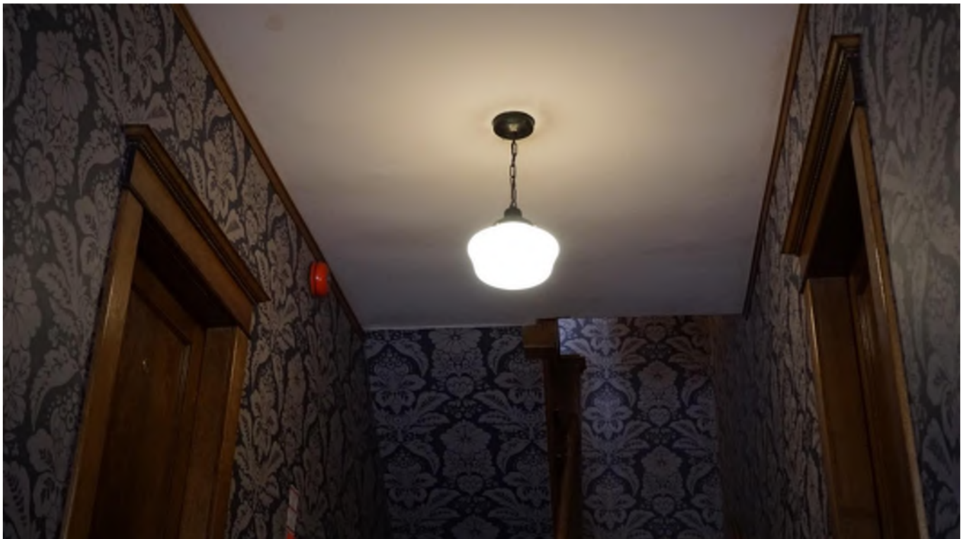
Figure 60 - Painted plaster ceiling and wallpapered walls.
