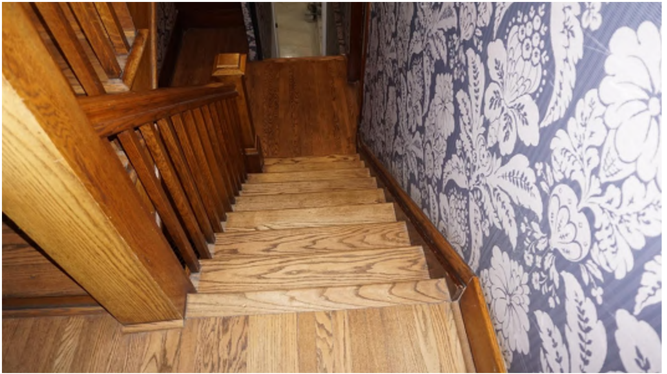
Figure 51 - View of the hardwood floor and stairs.
