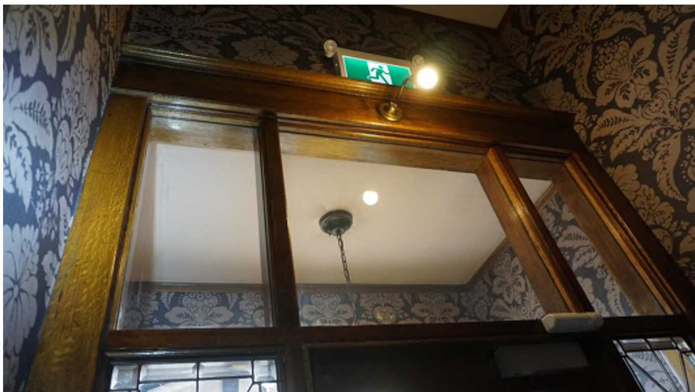
Figure 11 - View of woodwork detail of the inner vestibule.
