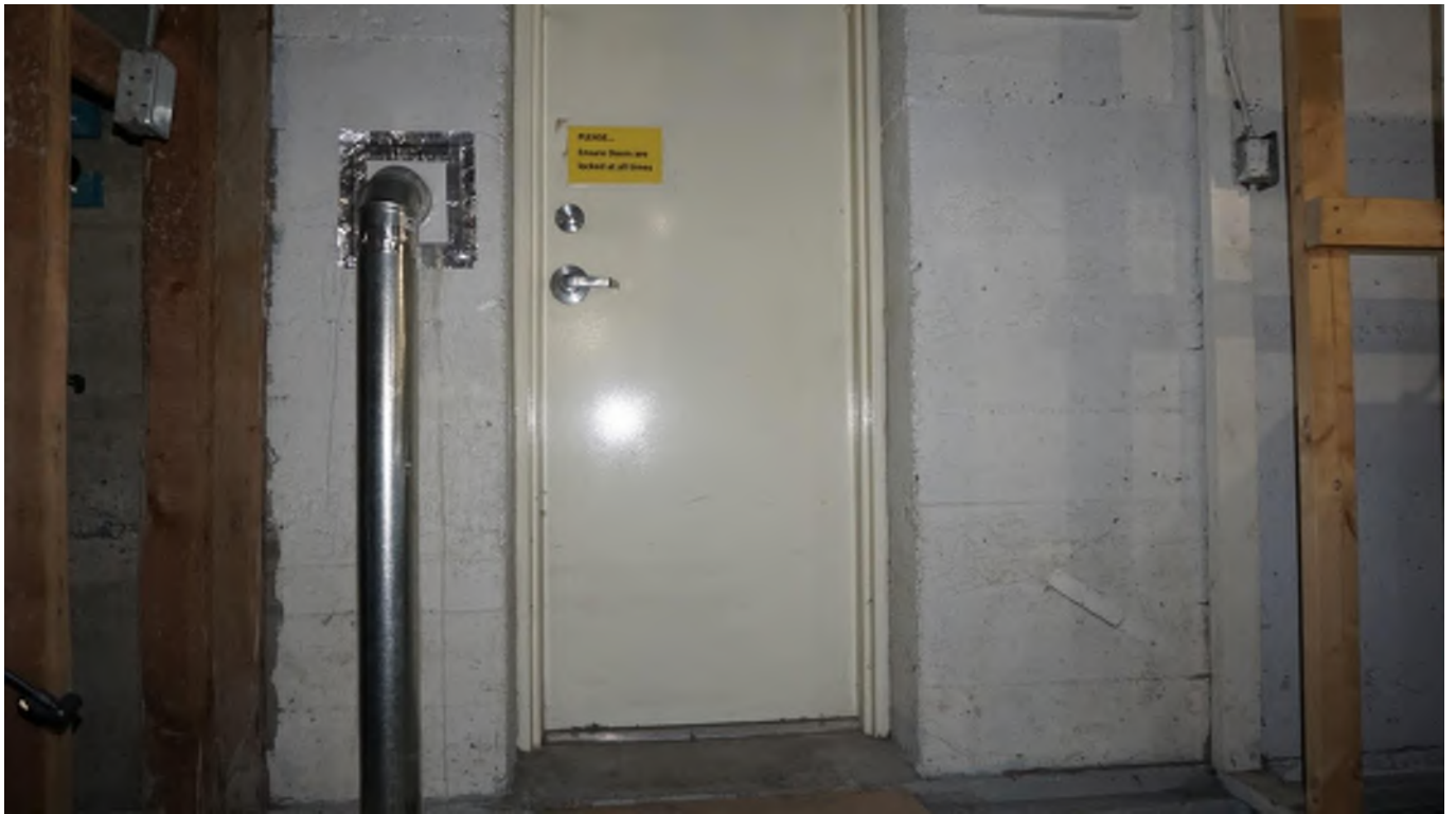
Figure 12 - Example of metal basement exit door.
