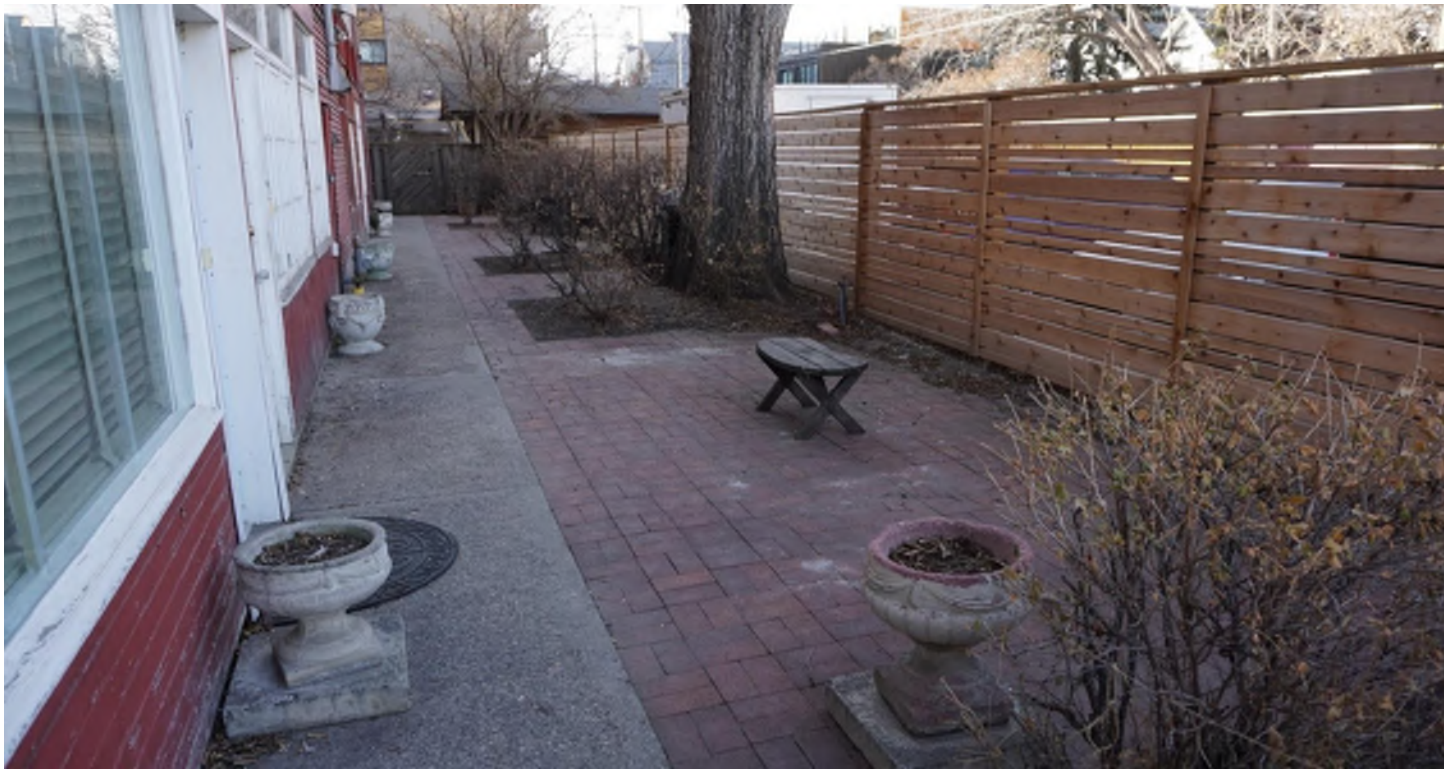
Figure 71 - Interlocking brick patios.
