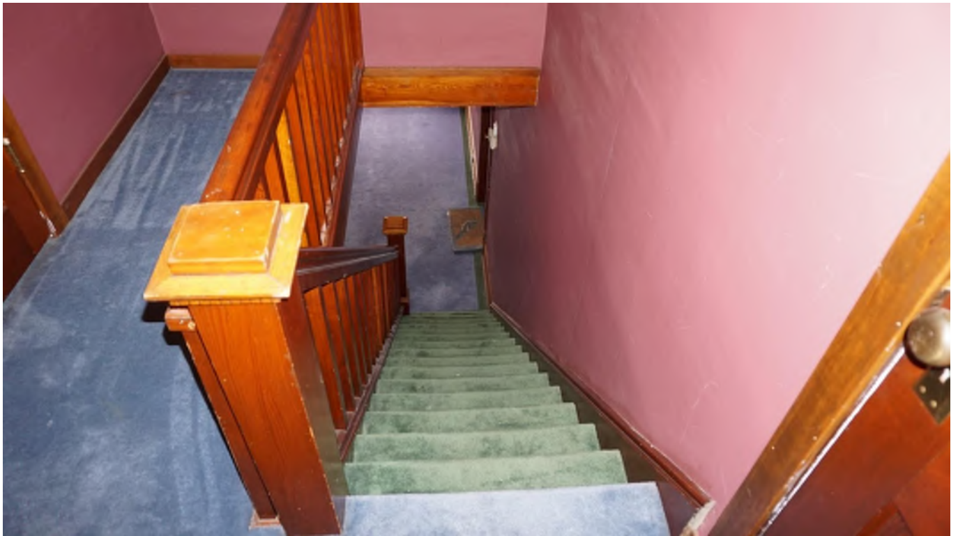
Figure 57 - Paint on the stairwell and landing to the attic floor in Building 908.
