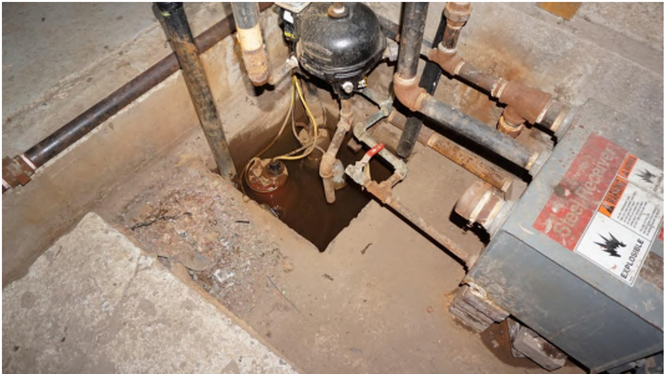
Figure 39 - Submersible sump pump.
