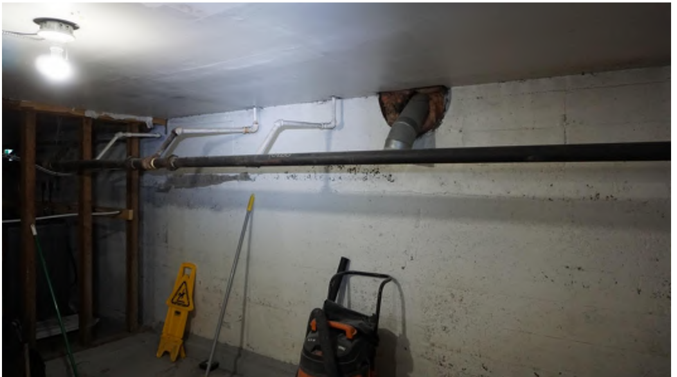
Figure 36 - Steel heating line.
