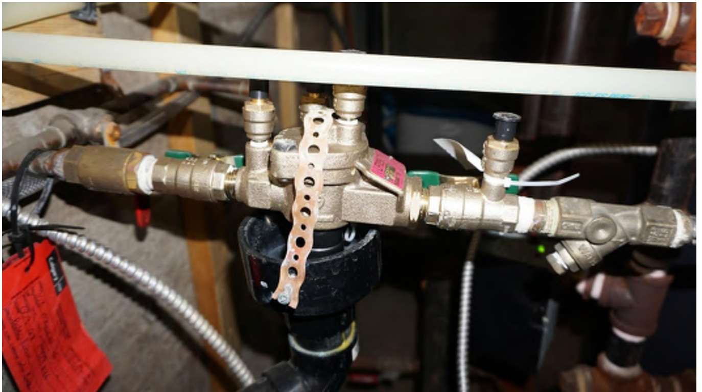
Figure 28 - Backflow prevention device.
