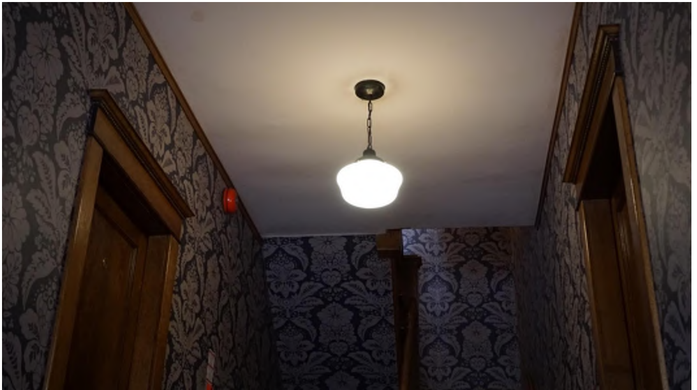
Figure 58 - 3rd floor ceiling.
