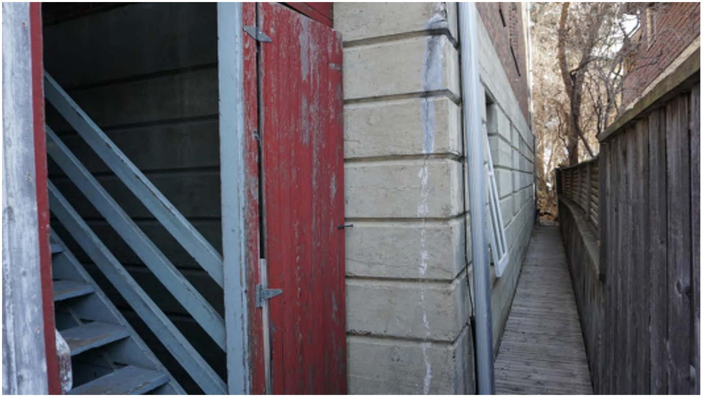
Figure 70 - Wood fence on west side.
