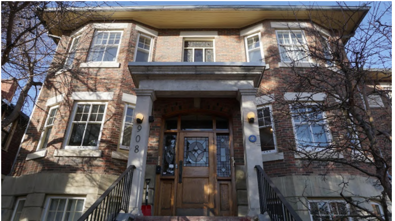
Figure 8 - Exterior view of the original hardwood doors with original hardware.
